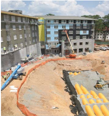
Few Hall &amp; construction of rainwater cistern
